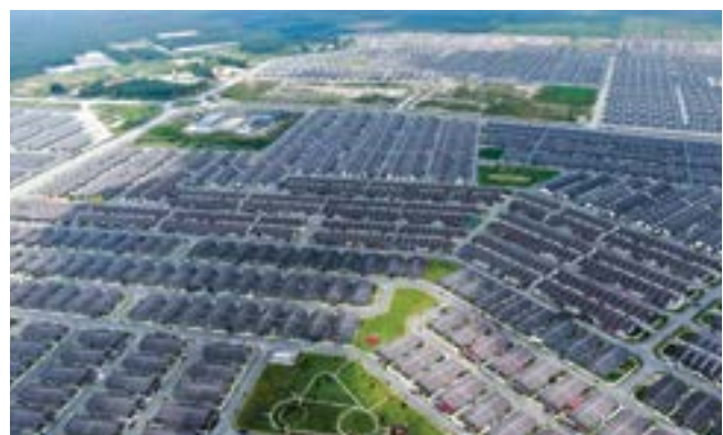
145,687 m 2 of landscape space created at BBSAP to promote rehabilitation and tree conservation
