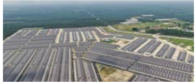
IBS application for BBSAP Phase 3A reduced construction waste generation
